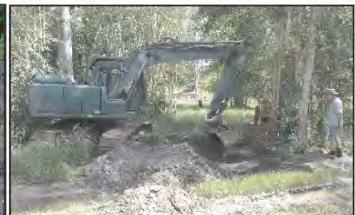
First drainage trench put in
